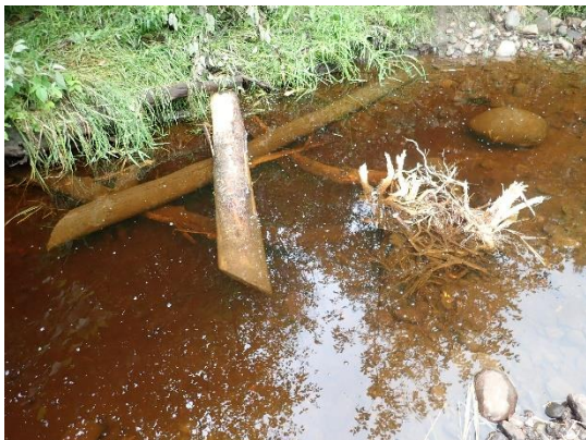
Complex wood habitat installed on Averill Creek. / Photo credit: Wisconsin DNR
