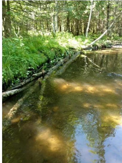
Log sill installed on N. Br. Beaver Creek./ Photo credit: Wisconsin DNR
