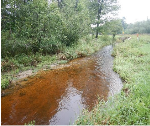
Riffle complex, post-installation on Bird Creek. / Photo credit: Wisconsin DNR
