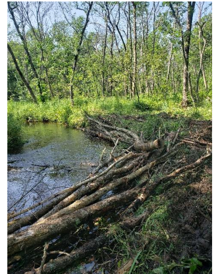
Log sill installed on Little Roche-A-Cri Creek. / Photo credit: Wisconsin DNR
