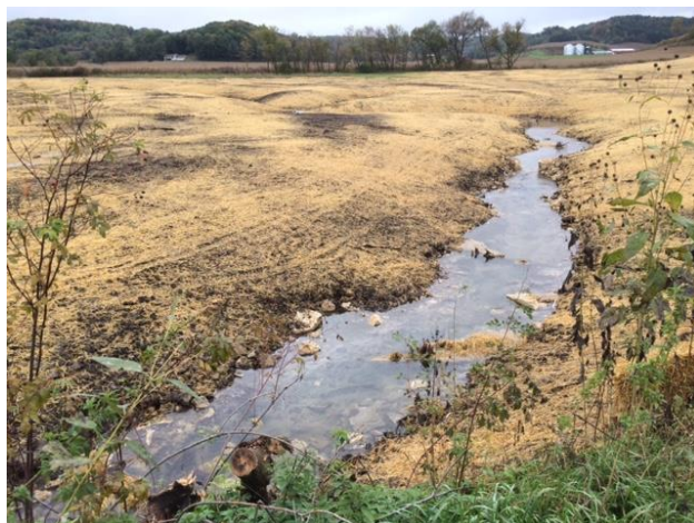
Hay Creek project area post habitat work. Streambanks were sloped and seeded to reconnect the floodplain with boulder clusters for instream habitat. / Photo credit: Wisconsin DNR
