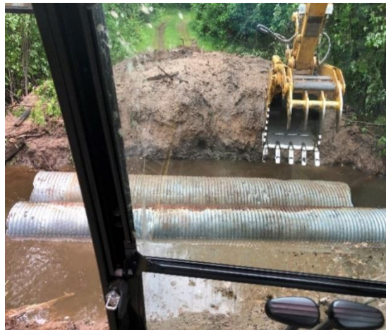
Left photo - Culverts being removed and reset. / Photo credit: Wisconsin DNR Right photo – The restored stream channel above the crossing after properly installing culvert. / Photo credit: Wisconsin DNR
