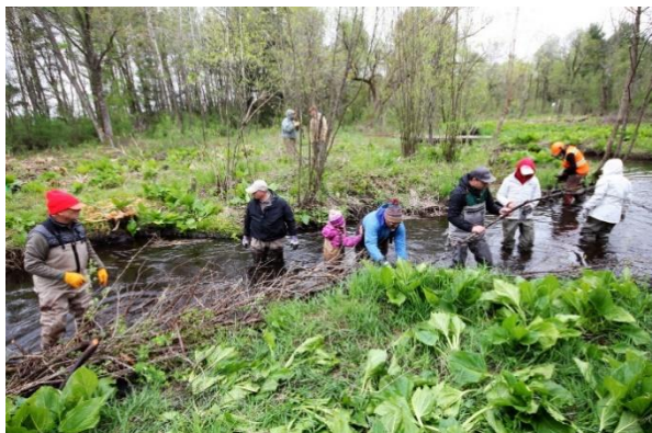
Volunteers working to install brush bundles and log sills on Bird Creek. / Photo credit: Wisconsin DNR
