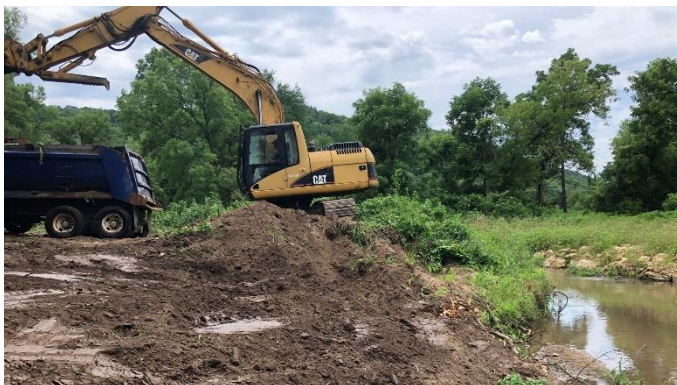
Left photo - Excavator removing deposition from the inside point to connect Rush Creek to floodplain. / Photo credit: Wisconsin DNR
