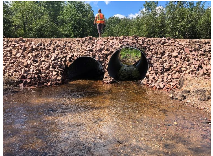
Newly installed culverts on Spring Creek. / Photo credit: Wisconsin DNR
