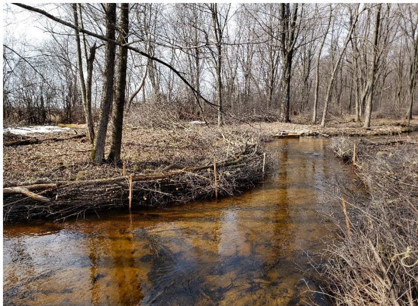
Plover River after riparian tag alder and buckthorn were removed and brush bundle/mattresses were installed. / Photo credit: Wisconsin DNR
