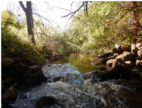
Mill dam site before project. / Photo credit: Wisconsin DNR
