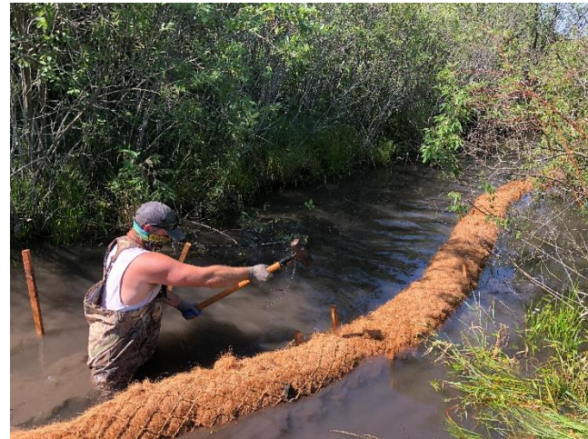
Installation of coconut fiber roll on Tichigan Creek to aid in narrowing stream channel. / Photo credit: Wisconsin DNR
