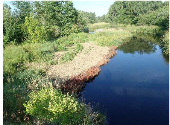
Brush bundles installed on the East Branch of the Eau Claire River. / Photo credit: Wisconsin DNR
