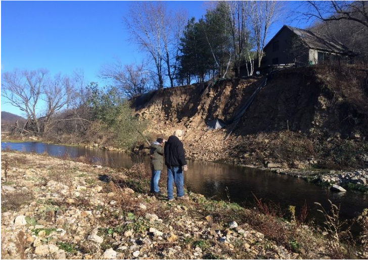
Eroding streambank, Frohock Creek, pre-project. / Photo credit: Wisconsin DNR
