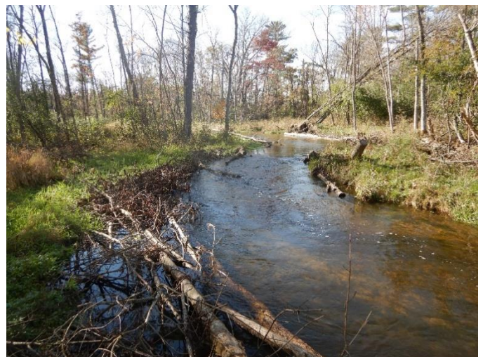
Log sill installation on the Pine River. / Photo credit: Wisconsin DNR
