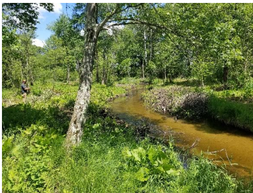
Brush bundles, log sills and fishability brushing completed on Bird Creek. / Photo credit: Wisconsin DNR
