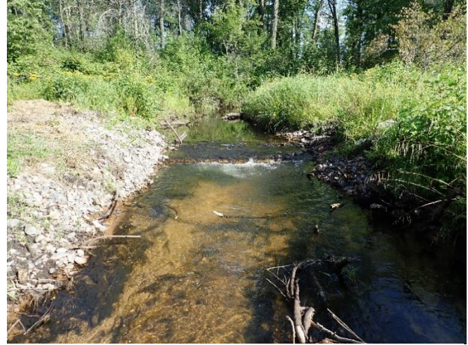
Plunge pool installed on Fordham Creek. / Photo credit: Wisconsin DNR
