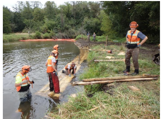
Bankcover installation / Photo credit: Wisconsin DNR
