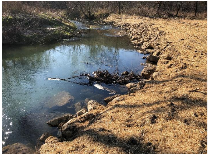
Same streambank completed with seed and mulch. / Photo credit: Wisconsin DNR
