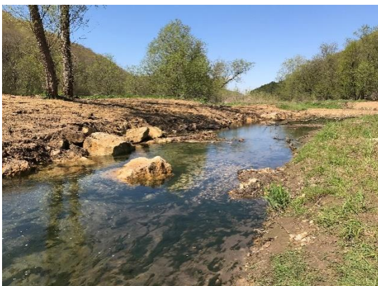
Streambanks along Sugar Creek immediately following completion of habitat work. Streambanks were sloped, seeded and stabilized with rock and root wads. / Photo credit: Wisconsin DNR
