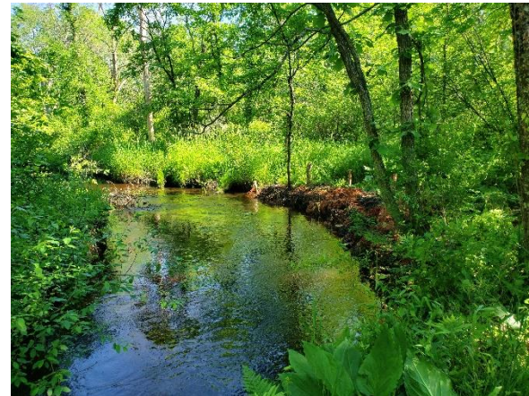
Brush bundles/mattresses installed on Little Roche-A-Cri Creek. / Photo credit: Wisconsin DNR
