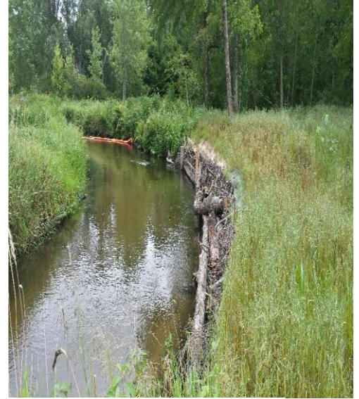
Log sill / Photo credit: Wisconsin DNR
