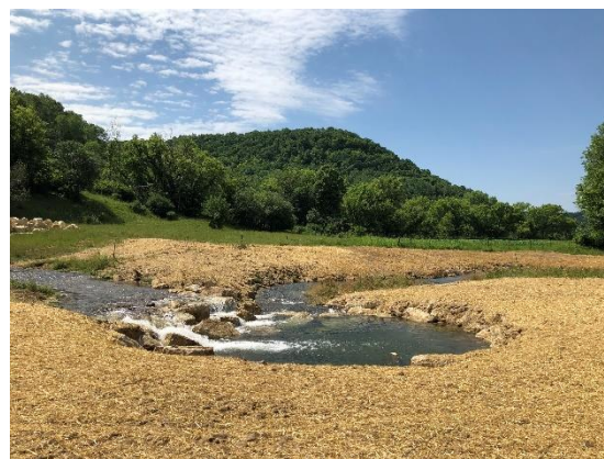
Recently installed rock weir with plunge pool on Coon Creek. / Photo credit: Wisconsin DNR
