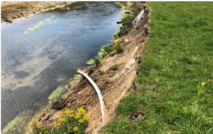
Left photo - Eroded streambank on Coon Creek with exposed drain field. / Photo credit: Wisconsin DNR
