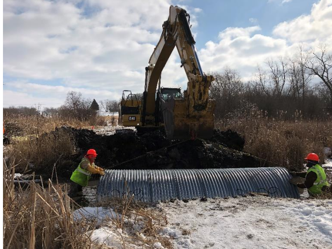
Installation of new culvert on Tichigan Creek. / Photo credit: Wisconsin DNR
