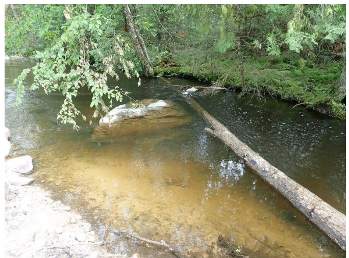
Large rock and large wood habitat installed on the Hunting River. / Photo credit: Wisconsin DNR
