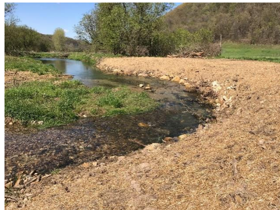
Streambanks along Sugar Creek immediately following completion of habitat work. Streambanks were sloped, seeded and stabilized with rock and root wads. / Photo credit: Wisconsin DNR
