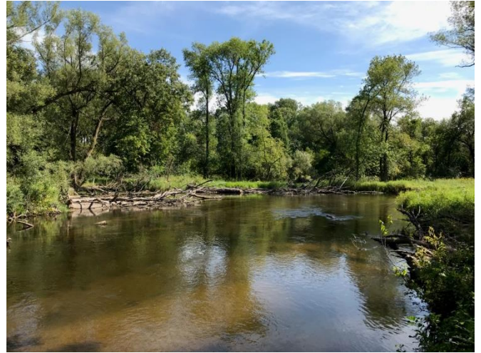
Log sills installed on Waupaca River. / Photo credit: Wisconsin DNR
